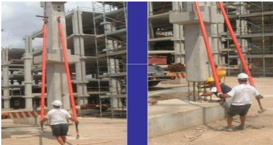
Fig. 1.2: Final Adjustment and Installation of Columns
