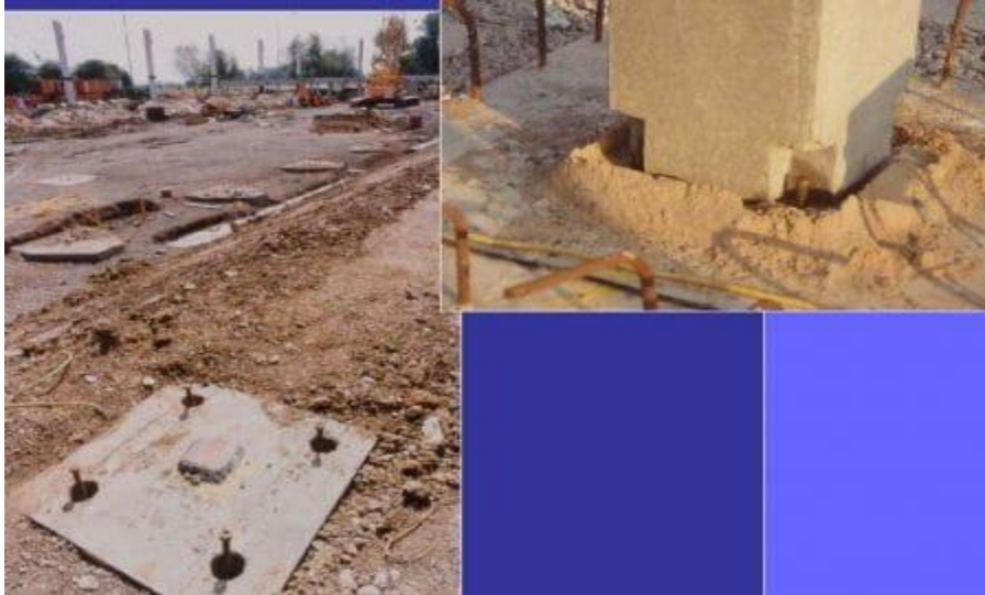
Fig. 1.1: Foundation for Precast Concrete Columns
