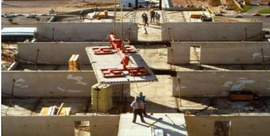
Fig. 1.6: Placement of Hollow Core Precast Concrete Slab on Walls
