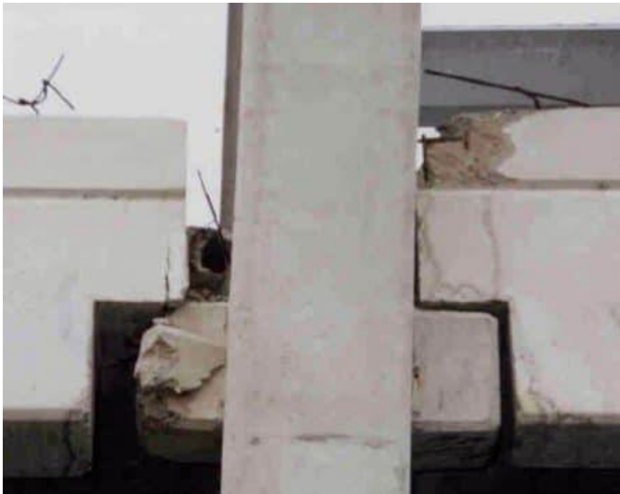
Fig. 2.9: Beam to Column Seated Connection
