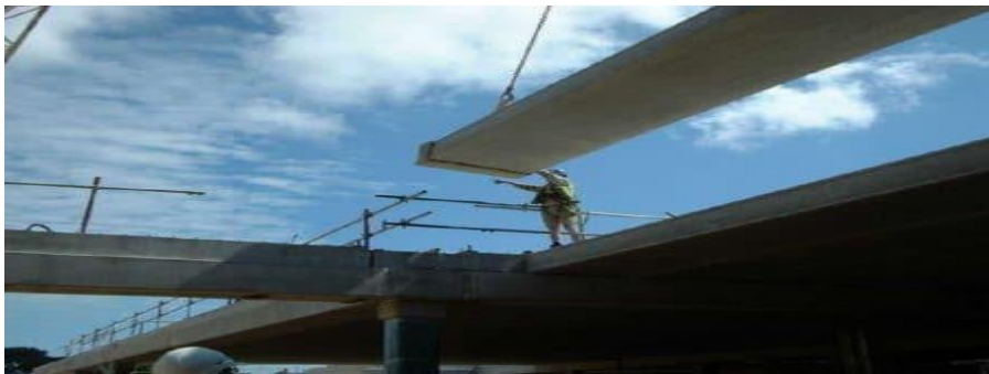
Fig. 1.7: Precast Concrete Slab Placement
