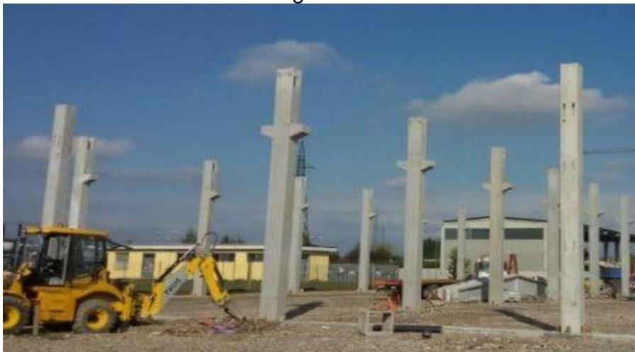
Fig. 2.5: Precast Concrete Columns
