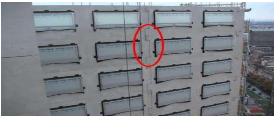
Fig. 2.12: Vertical Joint Using Deep Nib
