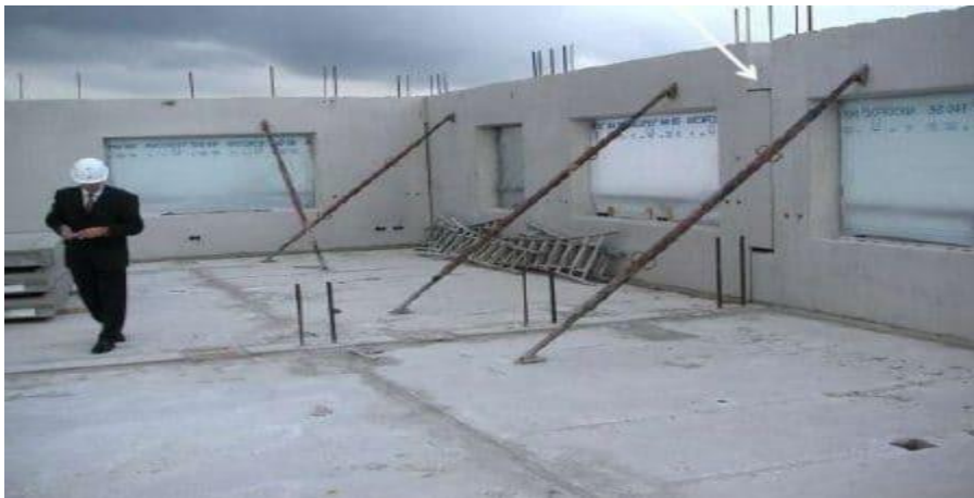
Fig. 2.11: Deep Nib Connection Between Walls Provide Large Complimentary Shear Stiffness and Strength
