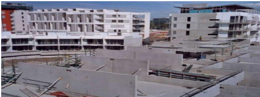
Fig. 1.4: Large Panel Precast Concrete System Construction
