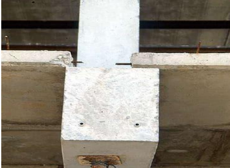
Fig. 2.10: Seated Connection
