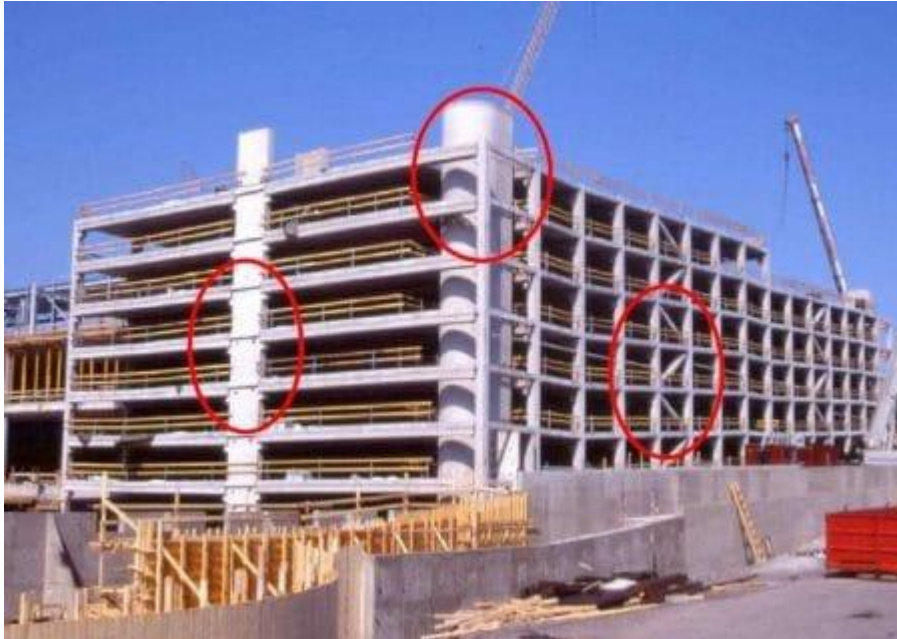
Fig. 2.13: Bracing Techniques
